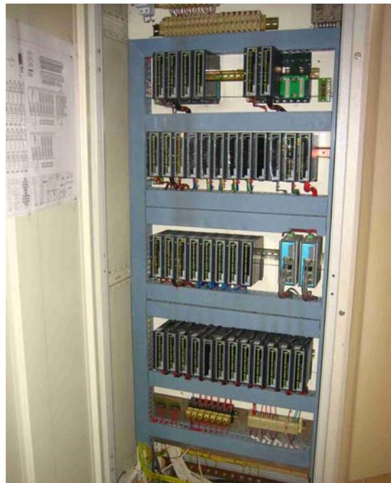
Fig.2: HSE Foundation Fieldbus controller's cabinet
