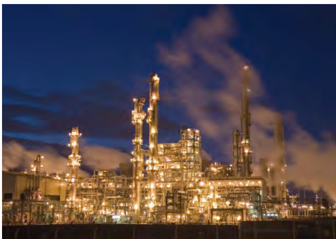
Fig. 1. Fieldbus technology is now replacing the traditional 4-20 mA platform as the basis for modern plant automation architecture
